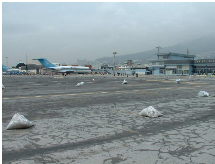
Figure 12 Ash was bagged in place then removed by truck.
