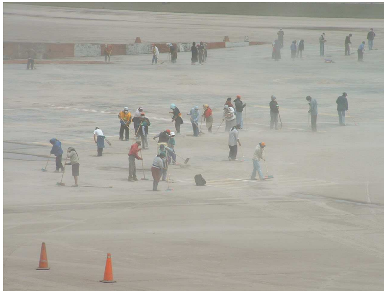
Figure 11 Five hundred workers took at least seven days to clear the runways with brooms, working for 15-hour shifts.
