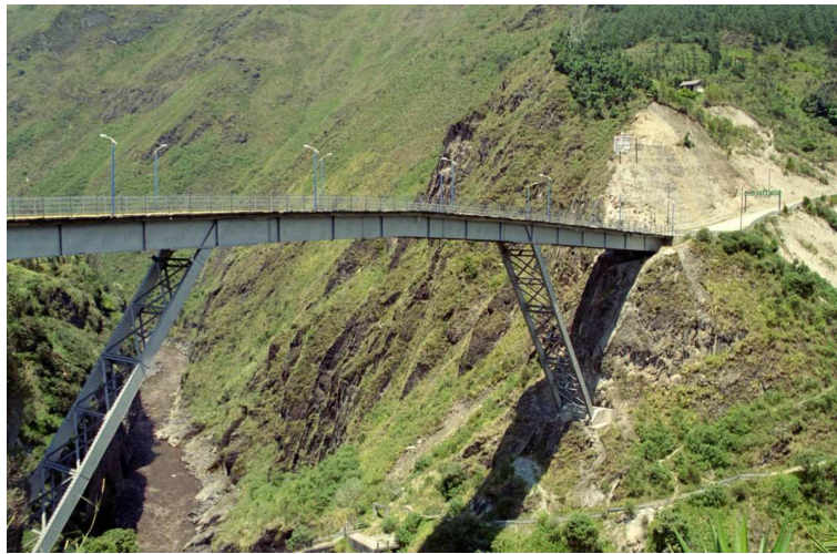
Figure 25 Bridge to safety: Installed since the 1999 reawakening of Tungurahua, this bridge provides an evacuation route from Baños (at left) but there is concern that it crosses the major lahar and pyroclastic flow valley, and connects to a part of Baños also likely to be in the path of a pyroclastic flow.
