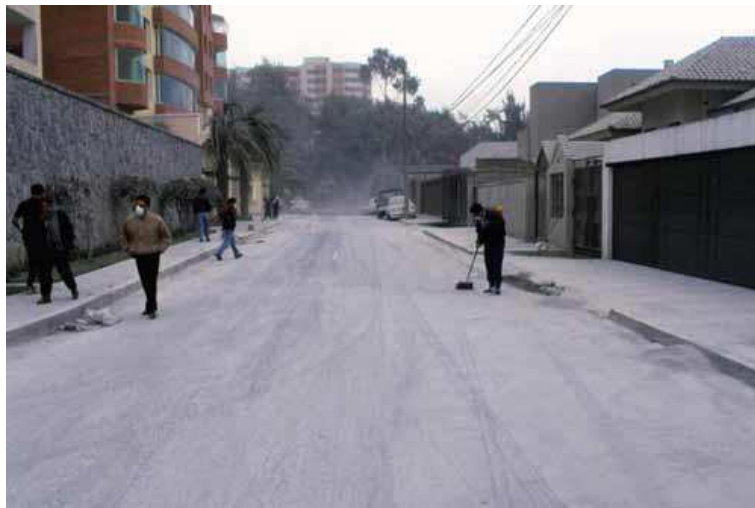
Figure 7 Streets are swept by hand in Quito, and ash enters storm water drains causing some blockage, but no damage to storm water pumps has been recorded. Ash is removed by trucks, so only a small proportion enters drains.
